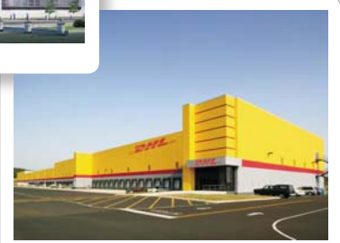
DHL Central Data Center
