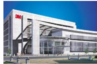
3M Central office, UK
